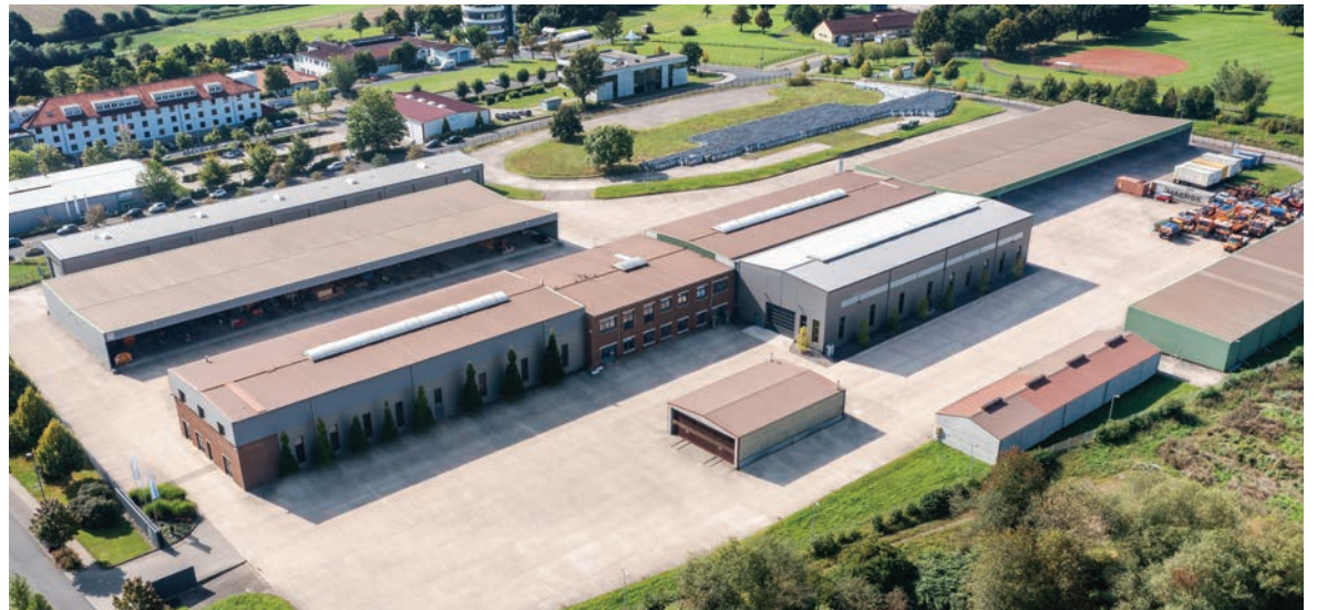
Uth GmbH, in the Muensterfeld region of Fulda, Germany, recently added a solar array to the roof of its 107,600-sq.-ft. assembly center. The photovoltaic system generates energy both for the company and the community of Fulda.
